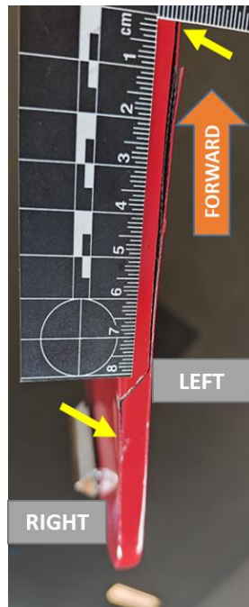
Figure 5 : underside view of the rudder crack
