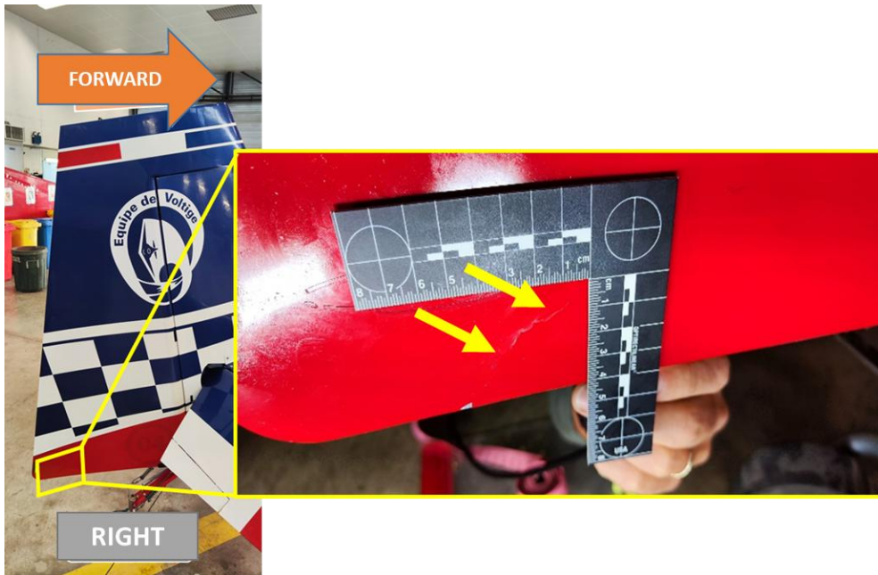
Figure 6 : crack on the right side of the rudder
